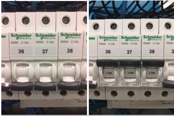
The circuit breaker on the left in the picture is in the OFF position, so that no electricity passes through it.
