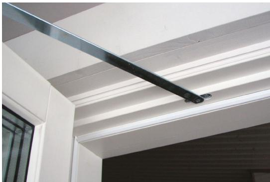
The venting hardware works using the door handle. Open the door to the desired ventilation position by turning the handle (diagram 1), which locks the door in position so wind gusts cannot slam it shut. If the handle is in the open position (diagram 2) the door moves freely.
