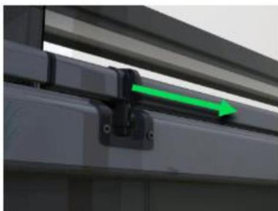
4. To close the glasses, do the opposite and finally lock the glass by pulling the gate wheel back into place.
