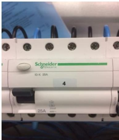
Figure: The RCD is in the I position and lowers the electrical circuit breakers and is ready to detect a possible fault in the electrical system.
