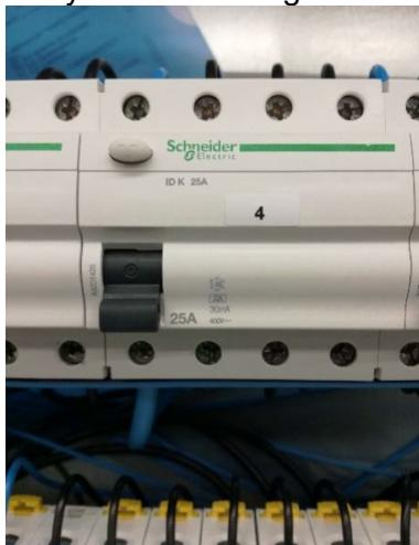
Figure: The RCD is in the O position. In this position, the RCD has operated and does not conduct electricity to the circuit breakers.
